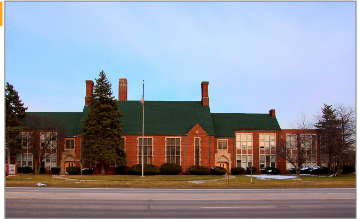
Originally the Annie Lathrup School, this is the last remaining historic structure on Southfield Road. This building is currently vacant.
